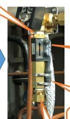
1. Disconnect the Flow switch from pipe line.
